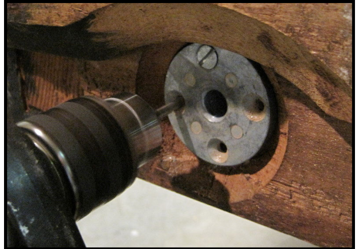
New socket being installed.
