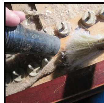
Removing the Debris
